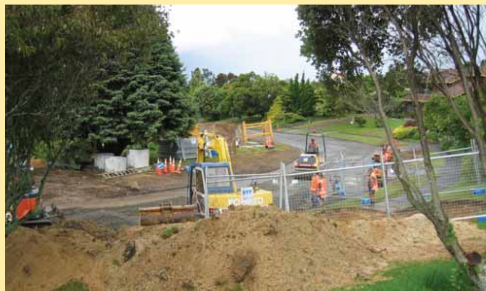
Works in Otarawairere are nearing completion.
