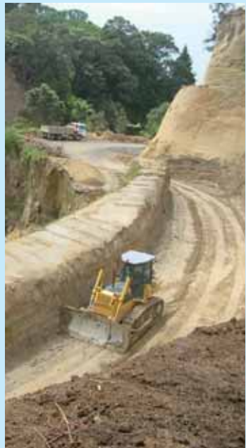
Herepuru Road under construction
