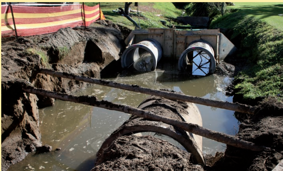
Hinemoa Drain Works
