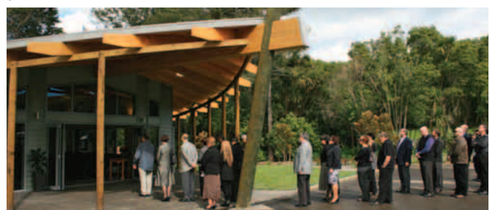
Whakatane Crematorium designed in the theme of a waka was officially opened in October 2009.
