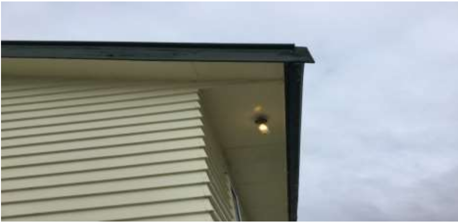
Soffit (Excluding Eastern Side)
