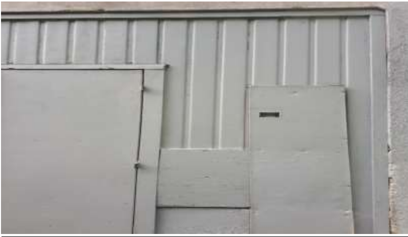
Exterior Cladding at Back Door
