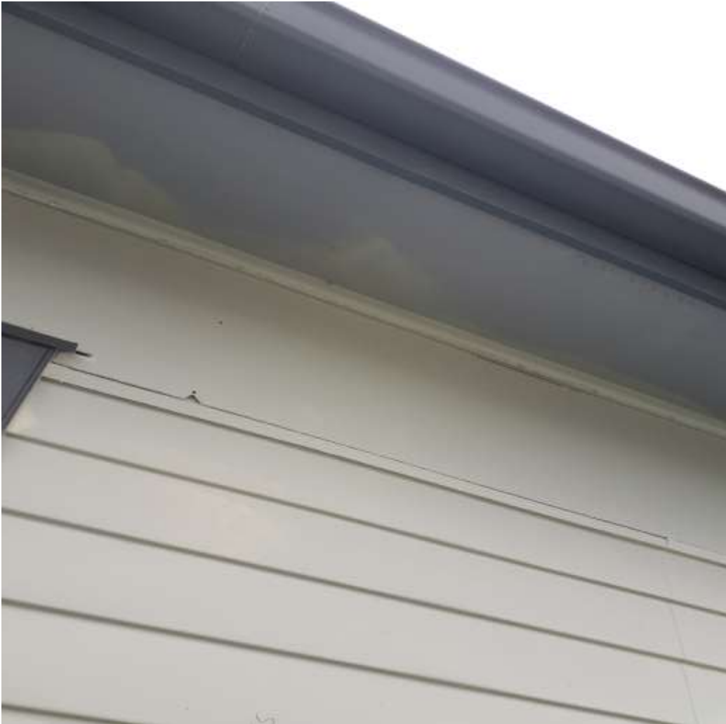
Soffit and Cladding (Top)
