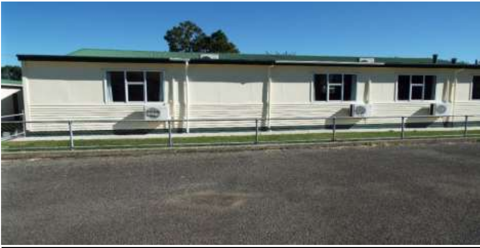
Cladding (Eastern Side)
