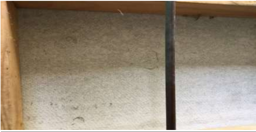
Internal Wall (from Service Room)
