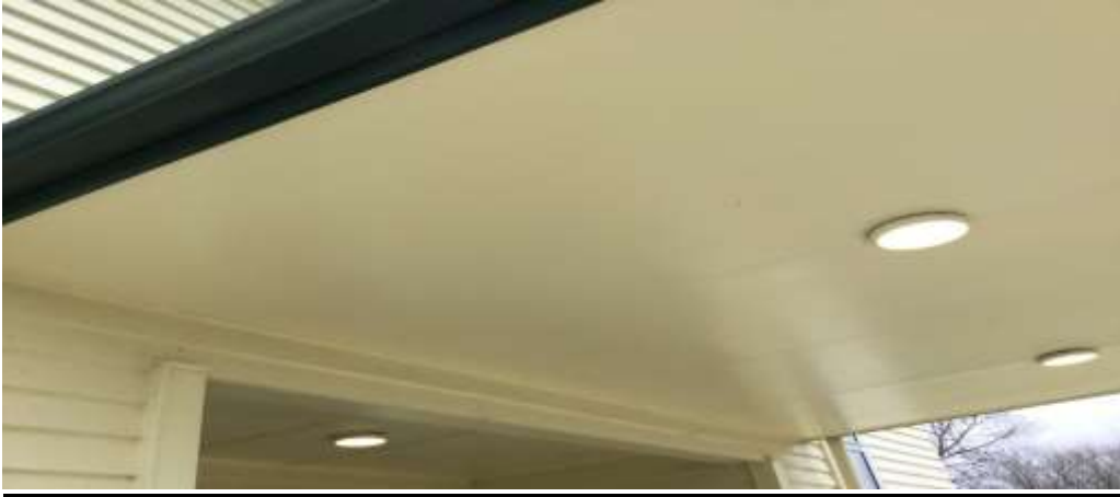
Entrance Canopy Ceiling
