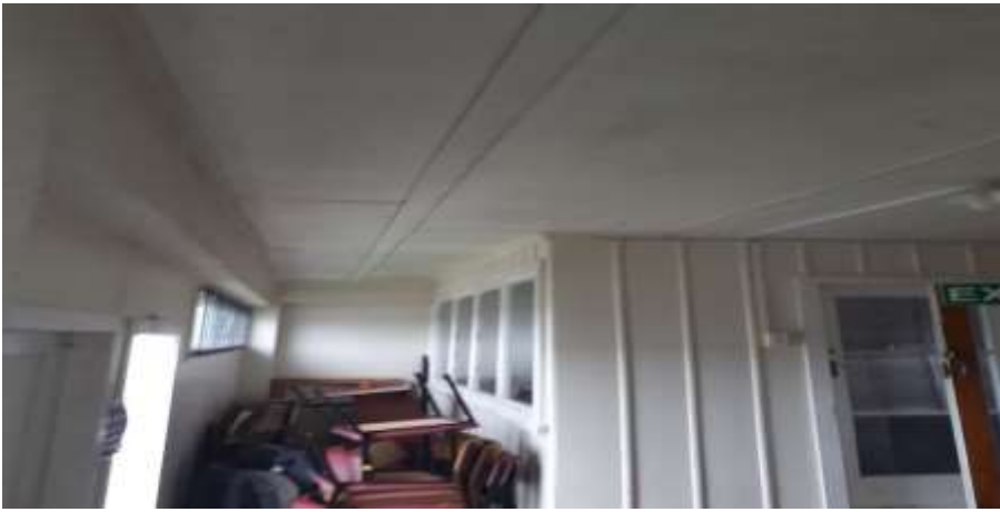
Entrance Ceiling and Walls
