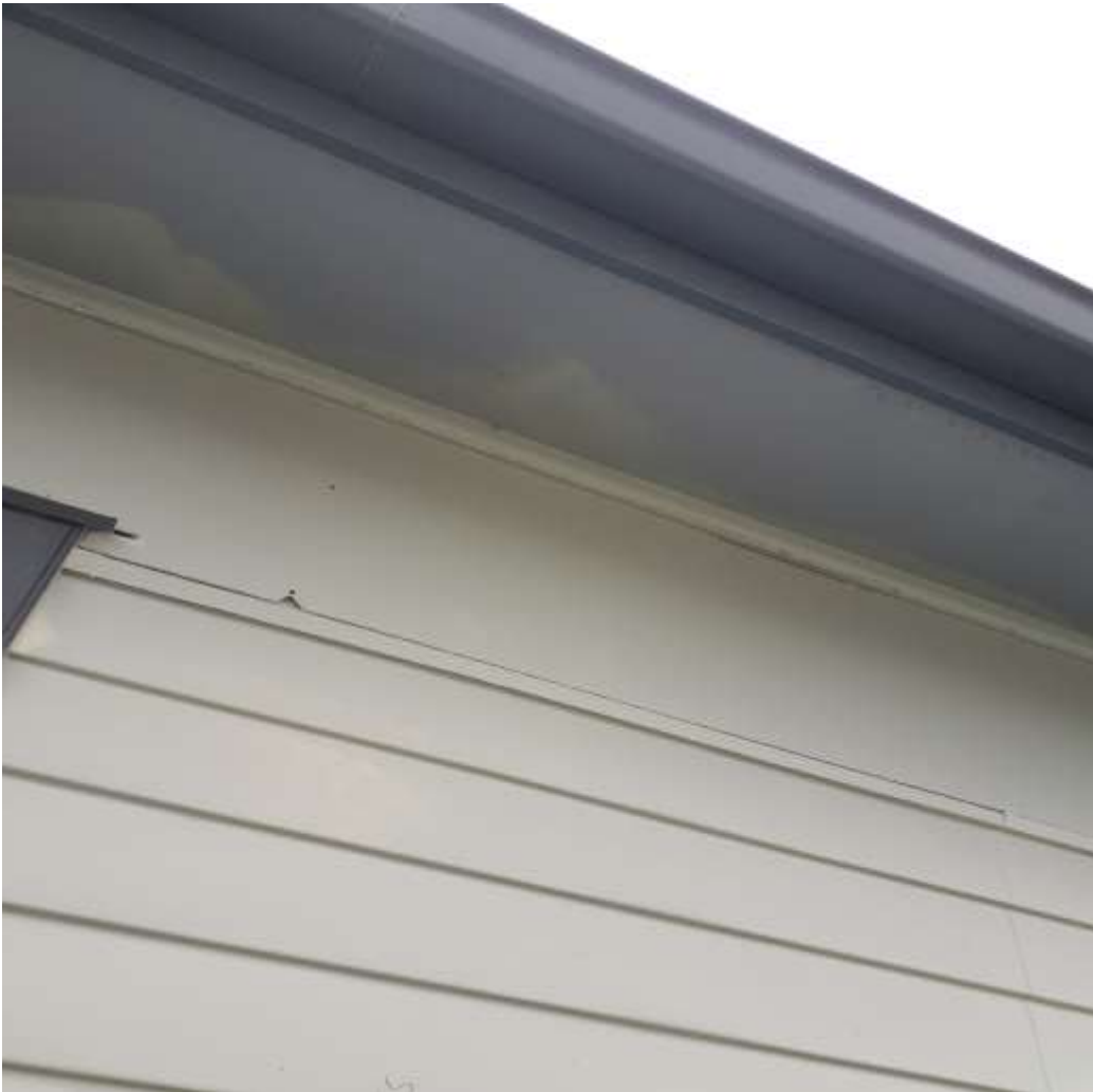
Soffit and Cladding (Top)
