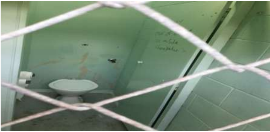
Internal Wall (from Toilet)
