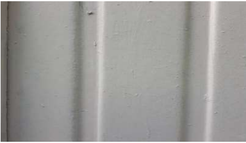
Exterior Cladding at Back Door
