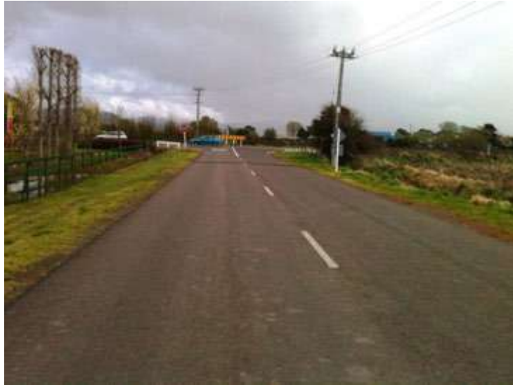
Photograph 2: Facing south on Huna Road toward SH30 with the site on the left
