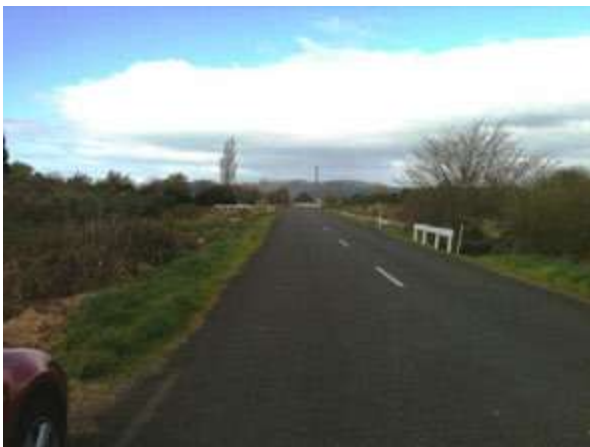
Photograph 3: Facing east on Kope Canal section of Shaw Road with the site on the left
