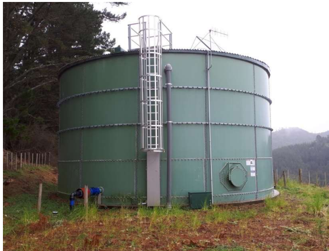
Figure 8: Steel Reservoir Constructed 2014
