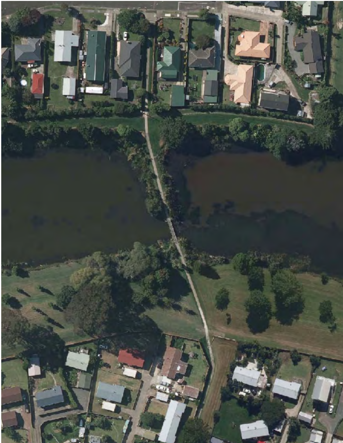
Figure 6: Direct route along the pedestrian causeway 6
