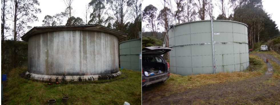
Figure 9: Concrete (Left) and Steel (Right) Storage Reservoirs
