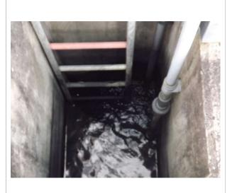
Figure 4. Polymer addition and slow mixing
