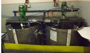
Figure 9. Bulk chemical storage THE P
