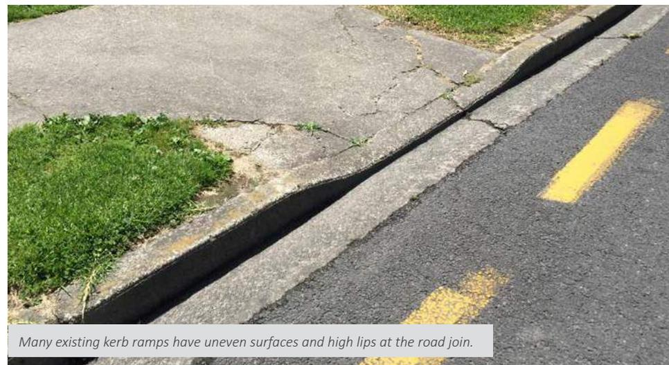
*Many existing kerb ramps have uneven surfaces and high lips at the road join.*
