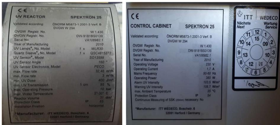
Figure 7: Ultra Violet Reactor and Cabinet Name Plates for Waimana
