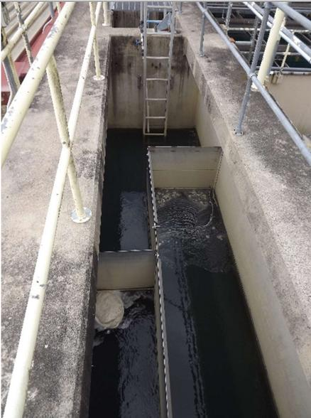
Figure 4. Polymer addition and slow mixing
