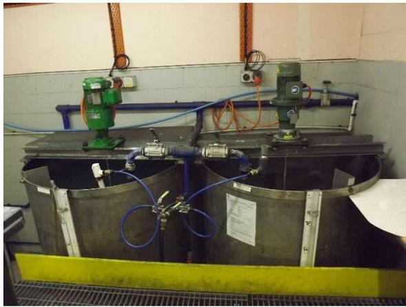
Figure 10. Polymer makeup tanks
