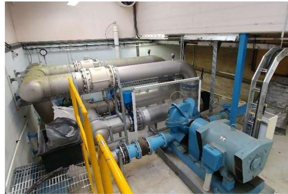
Figure 11. UV Reactors and High Lift Pumps
