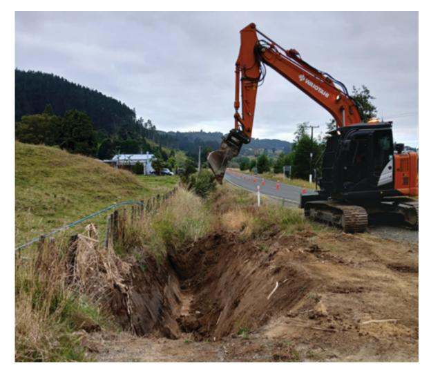
A previously buried 900mm diameter stormwater culvert on SH2, near the entrance to the Tāneatua reservoir, was recently discovered. Work is now underway to uncover and reinstate the culvert, which is expected to provide significant relief to the stormwater drainage that affects the eastern side of Tāneatua township during heavy rainfall events.
