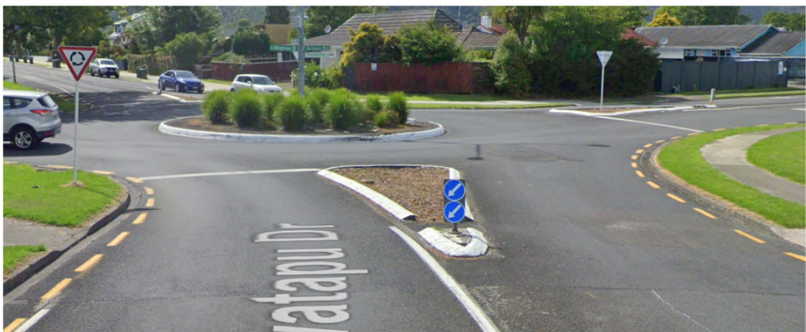
Figure 1 - Narrow islands on the roundabout approaches do not provide enough space for pedestrians to wait for gaps in traffic.
