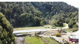
A staged approach will be used for the bridge opening expected to begin in early April which will see the traffic lane opened first. This will allow for the temporary bridge to be demolished and the fill from the approaches used for the permanent road. Earthworks are well under way and the approaches are being constructed using cut and old slip material.
