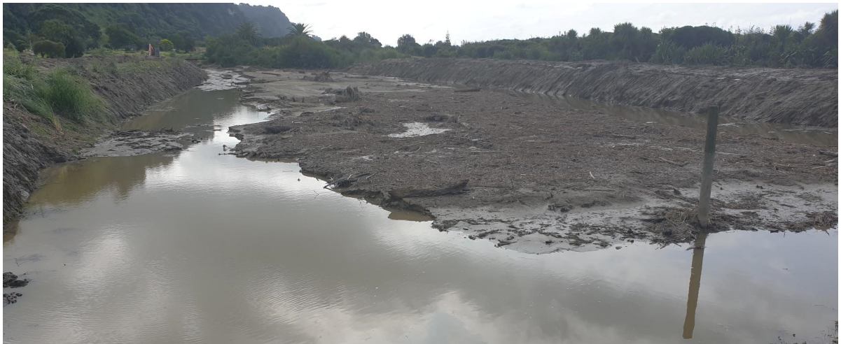
Awatarariki primary sediment pond during initial cleanup following 4 February 2025 storm event.
