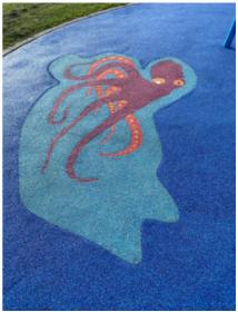
The Ocean Playground safety surface replacement has been successfully completed, following the installation of a new rubber 'pour and play' surface that addresses deteriorating conditions and eliminates the need for ongoing patch repairs around high-use areas like the swings.
