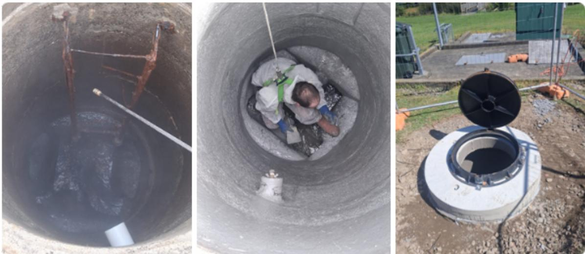
Forty-three key receiving manholes across the Whakatāne, Ōhope, and Edgecumbe wastewater schemes have been inspected as part of condition assessment activities. The inspections confirmed that the manholes are in poor condition, with varying levels of corrosion requiring refurbishment to prevent further deterioration.
