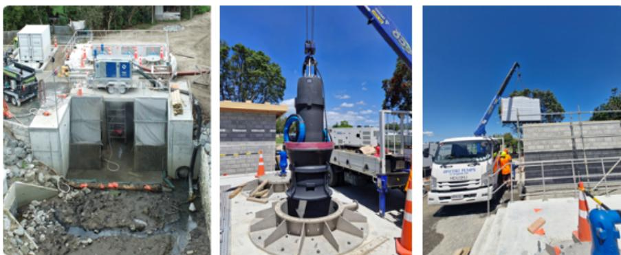
Construction of the Hinemoa stormwater pump station is nearing completion. The concrete quality issues identified in the pump station roof slab have been remedied by Construction Technologies, an Auckland-based specialist in concrete repair and maintenance. The cost of these remedial works has been deducted from the contractor's contract price.
