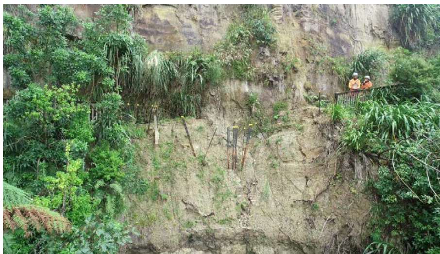
Figure 3 (2024): Landslide 2 – an underslip where most surface material has slid off exposing the sandstone underneath.
