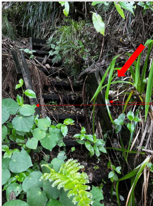
Photo 18: Old track above the current alignment to the north of slip 1. The hand rails are being 'squeezed' by the colluvium that is moving down the slope.
