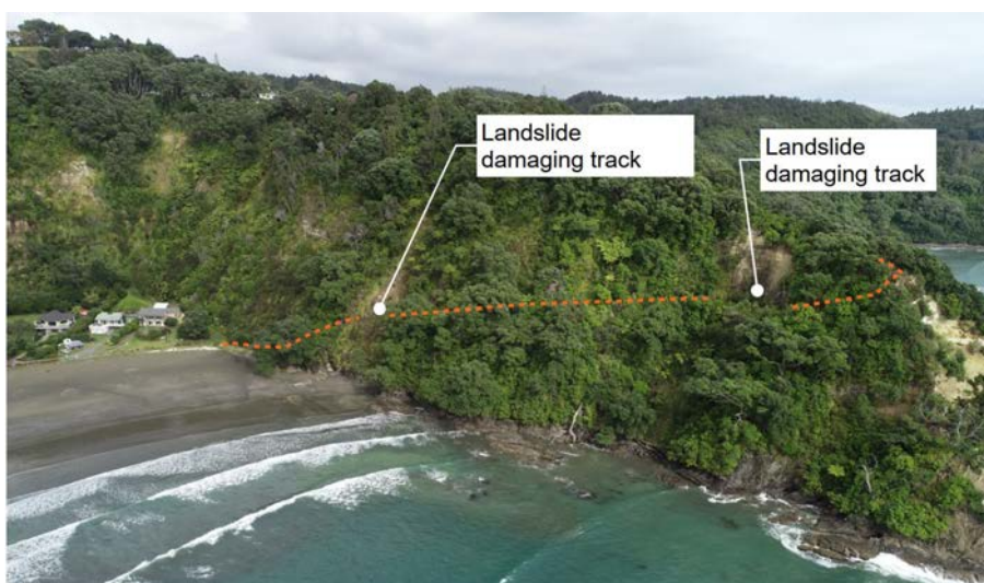
Figure 1.1: Two recent landslides damaging the existing track.
