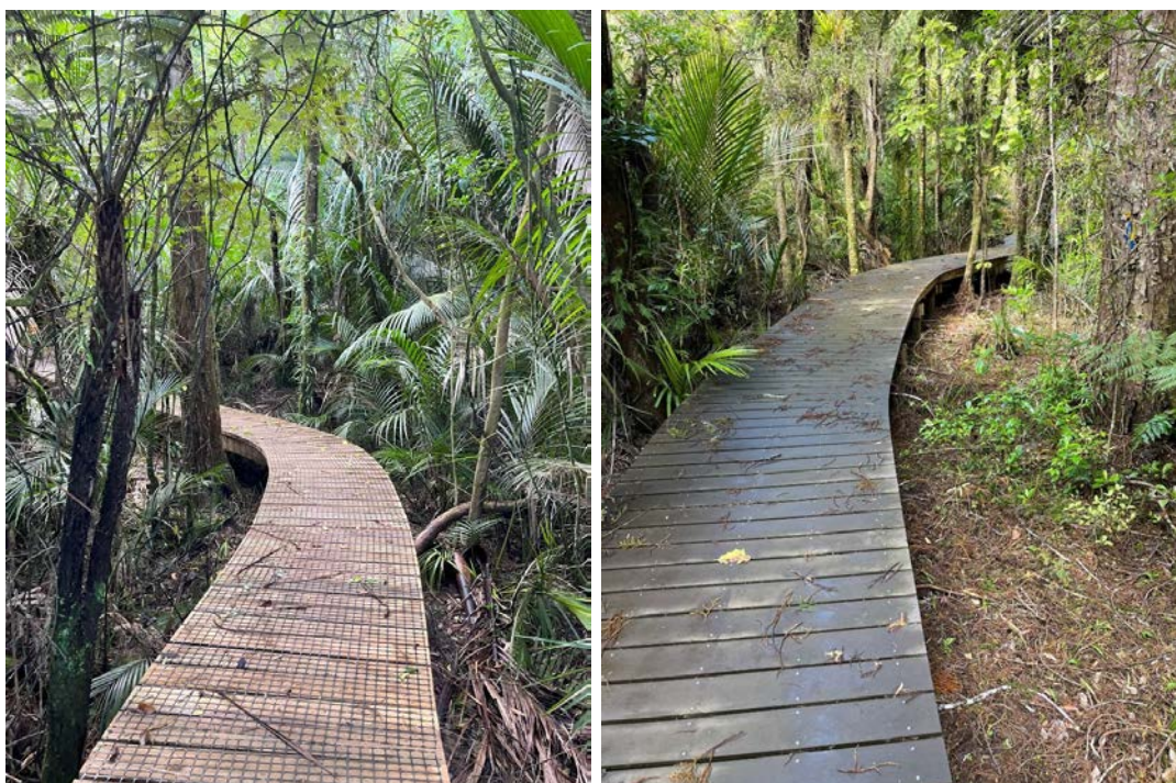
Figure 9 & 10: Boardwalk across wet areas where natural hydrology is to be maintained
