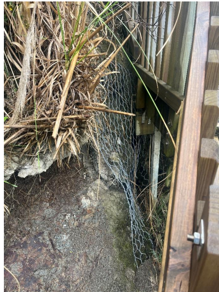
Photo 2: Staircase with mesh around foundation location
