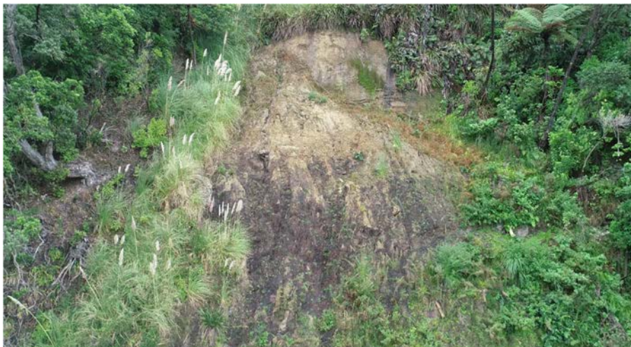
Figure 2 (2024): Upper section of landslide 1.
