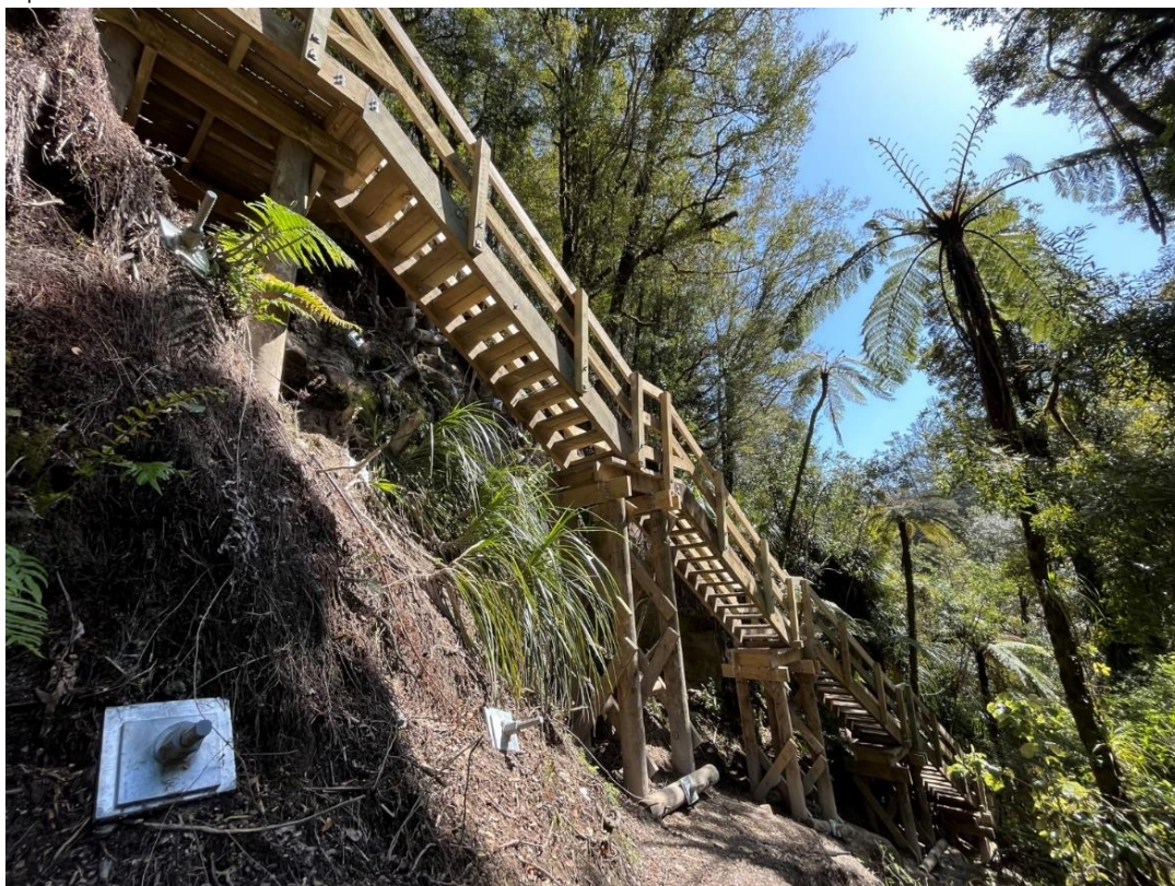
Figure 2: Similar staircase up steep rock face on Omanawa Falls Track
