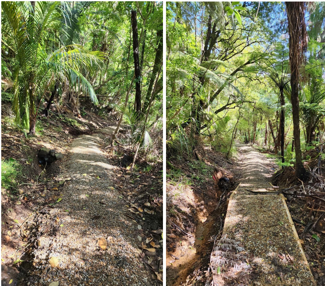
Figure 11 & 12: Typical aggregate track in bush setting with occasional small flights of boxed steps
