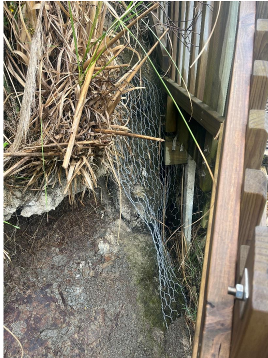
Figure 5: Localised rock mesh above foundations to protect structure.
