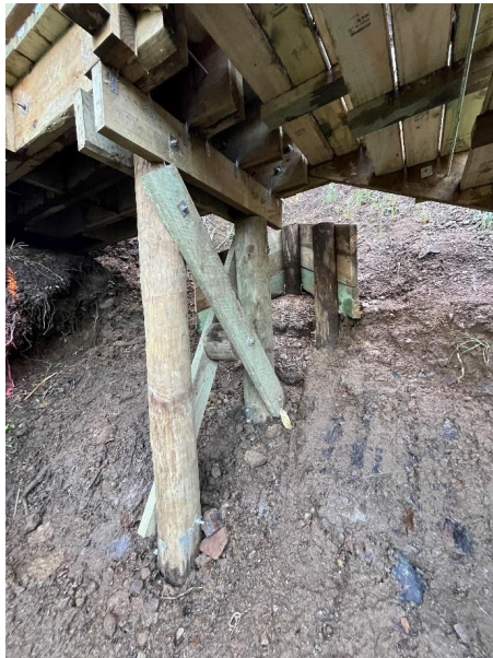
Photo 1: Deflector to protect structure foundations over slip
