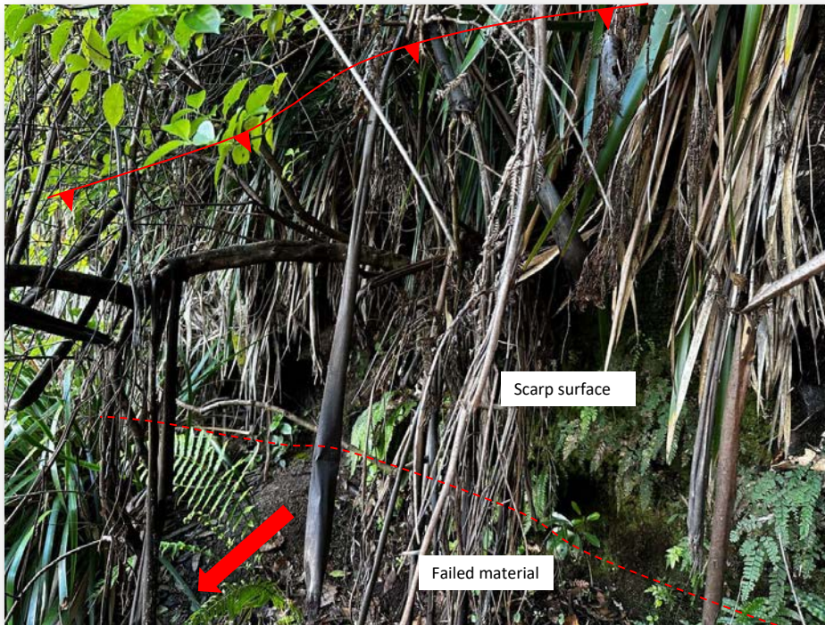
Photo 7: Head scarp 1. Looking south.
