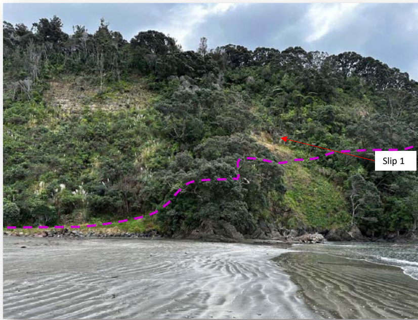
Photo 1: Looking up at 'slip 1'. Approx original track alignment shown by pink line.
