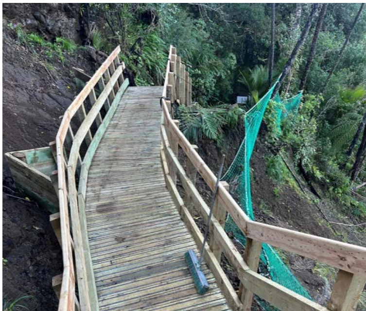
Figure 4: Boardwalk across slip face with deflectors at foundation locations
