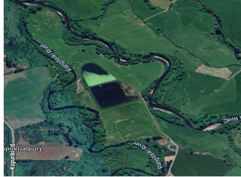
Murupara Wastewater Treatment Plant Location
