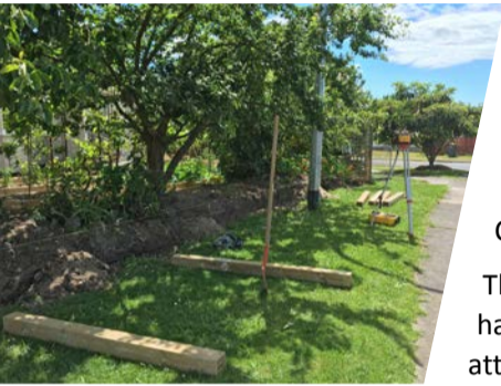
Preliminary work is underway for Sunday's fence-building workshop.
