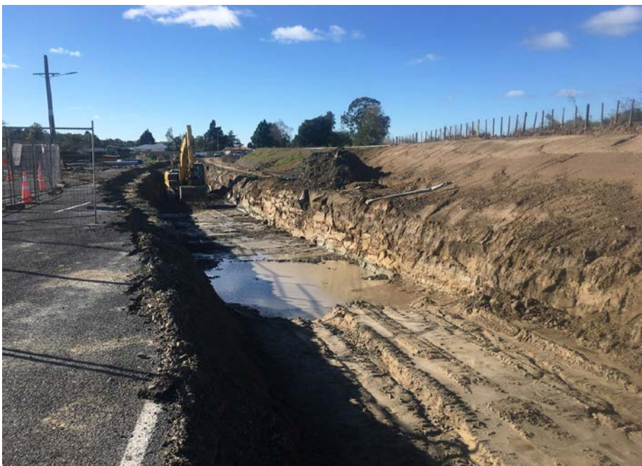
Good progress reported on the College Road stopbank works.
