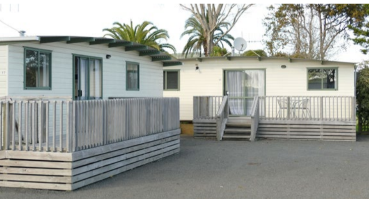
Ten new two-bedroom, fully self-contained relocatable units similar to these existing units at the Whakatāne Domain Holiday Park will soon be available for temporary accommodation.
