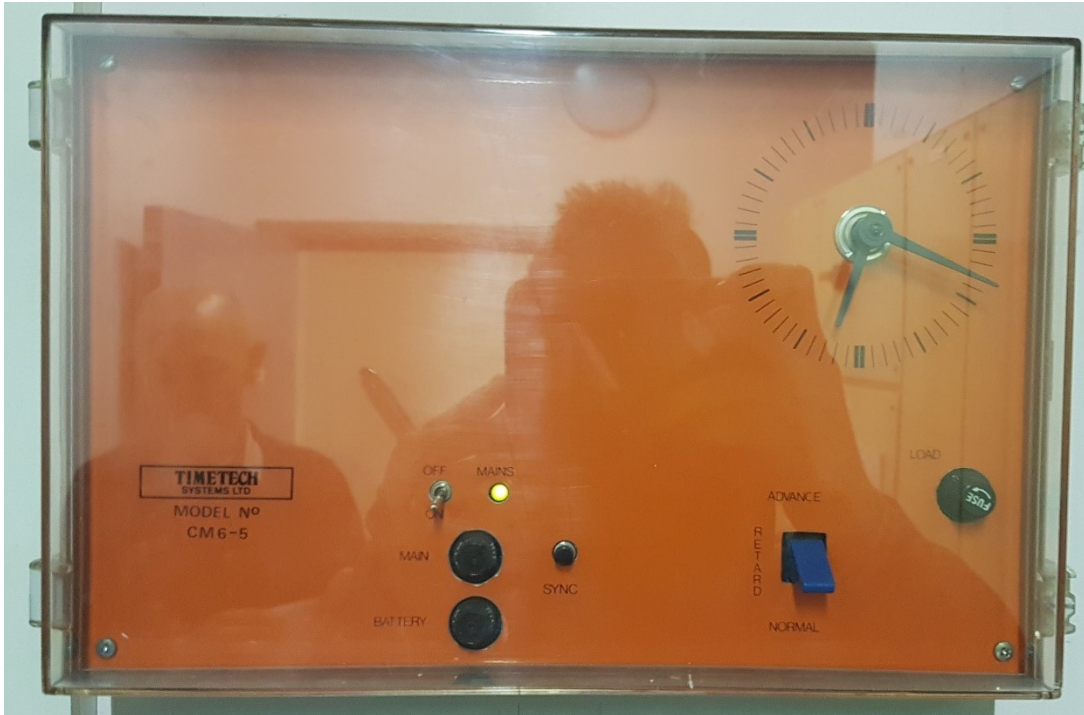
Figure 8-5 - Time based building services control system
